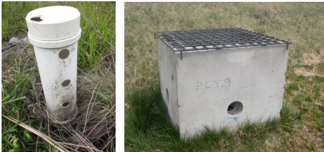
Outlet structures designed for peak flow mitigation in Camp Pendleton, California (left), where a graduated riser pipe regulates drawdown of the detention volume, and (right) at Southwest Middle School in Gastonia, North Carolina, where orifices allow controlled dewatering of the detention volume—the water quality treatment volume is retained below the orifice elevation.
