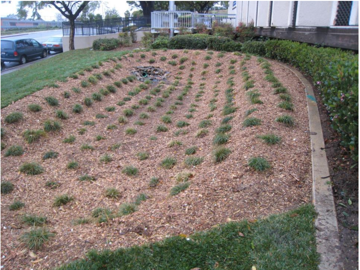
Figure A.1-1. Bioretention in landscaped area.
